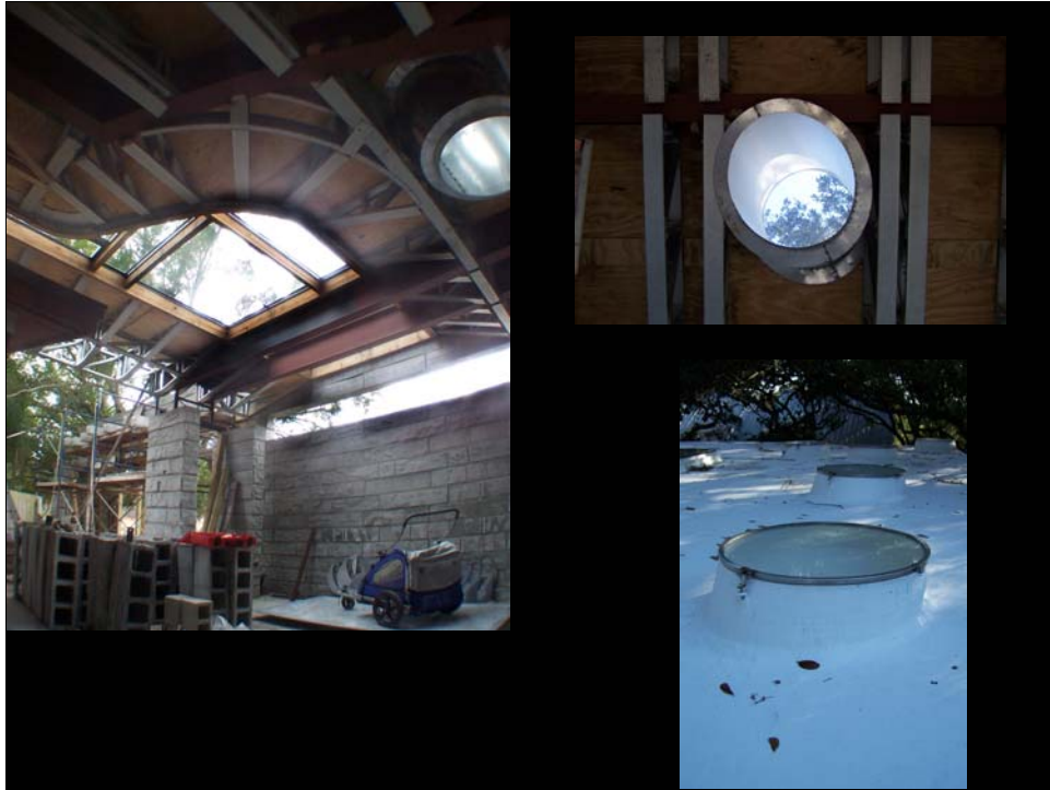
Photos of installed skylights. The roof at lower right is a fluid applied acrylic membrane. This one is by Hydrostop® www.hydrostop.com .
