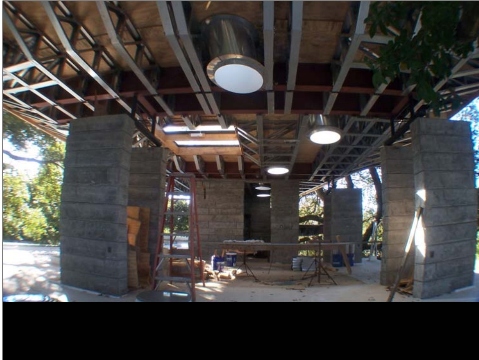
Skylights beginning to define the quality of light in the space.
