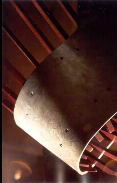
¼" Aluminum structural plate, steel base. Hardwood (purpleheart) ribs attached with countersunk SS screws.
