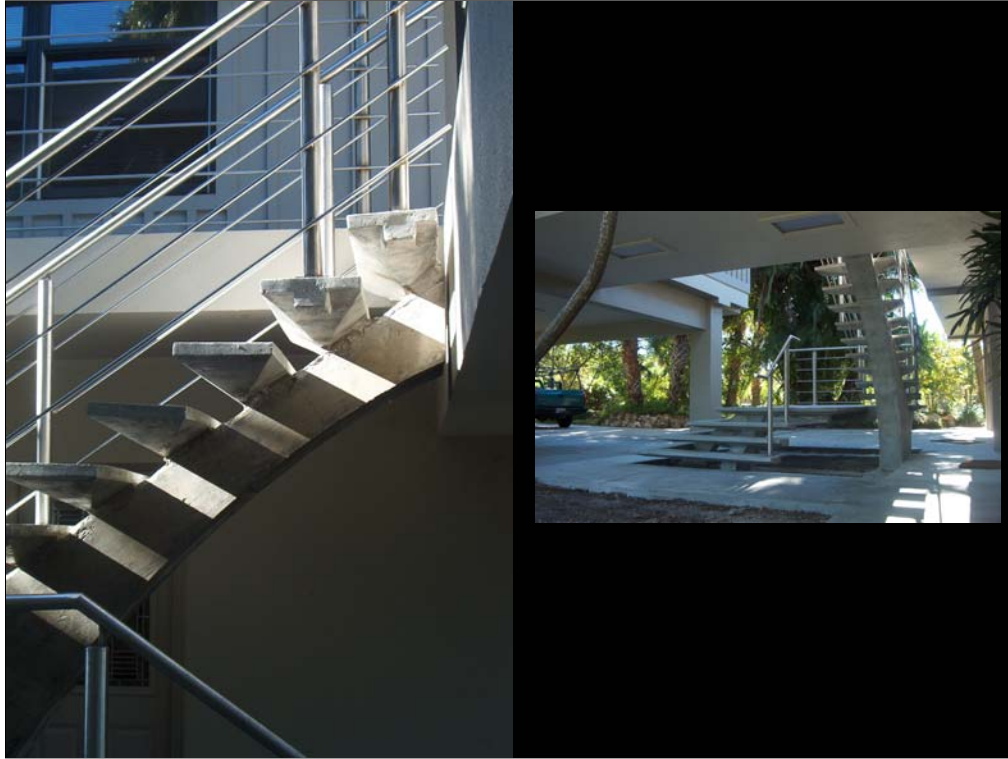
Cantilever, independent structure.
