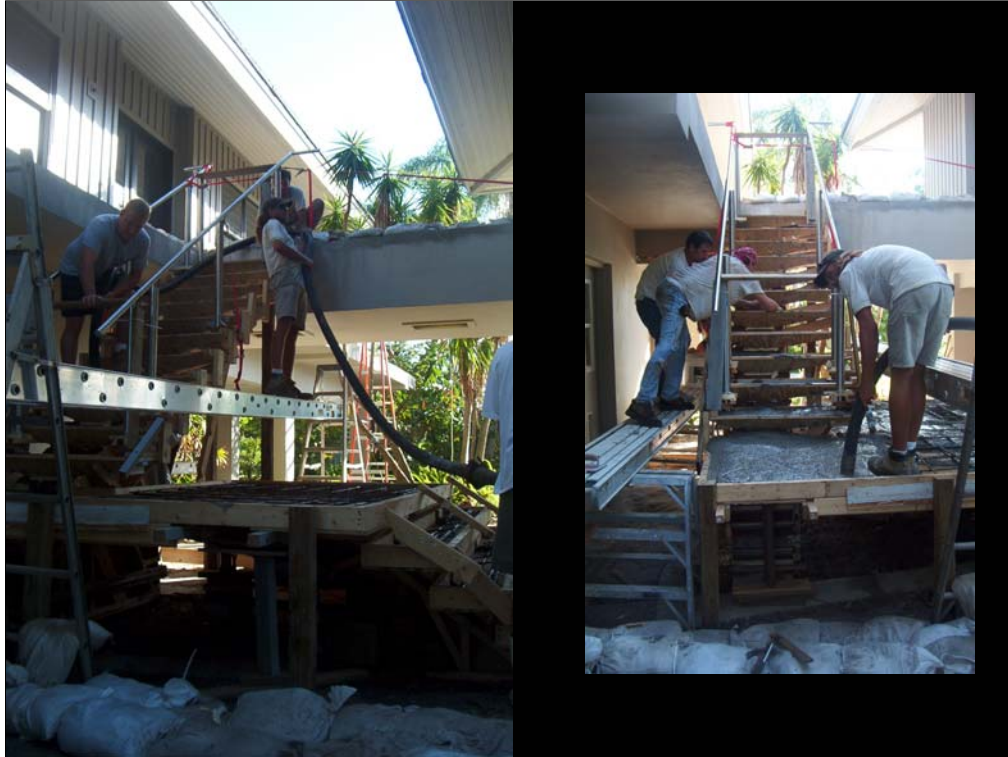
Left, filling the holes between layers. Right, the lower treads have set up enough to resist the pressure and the pour can continue for the moment.
