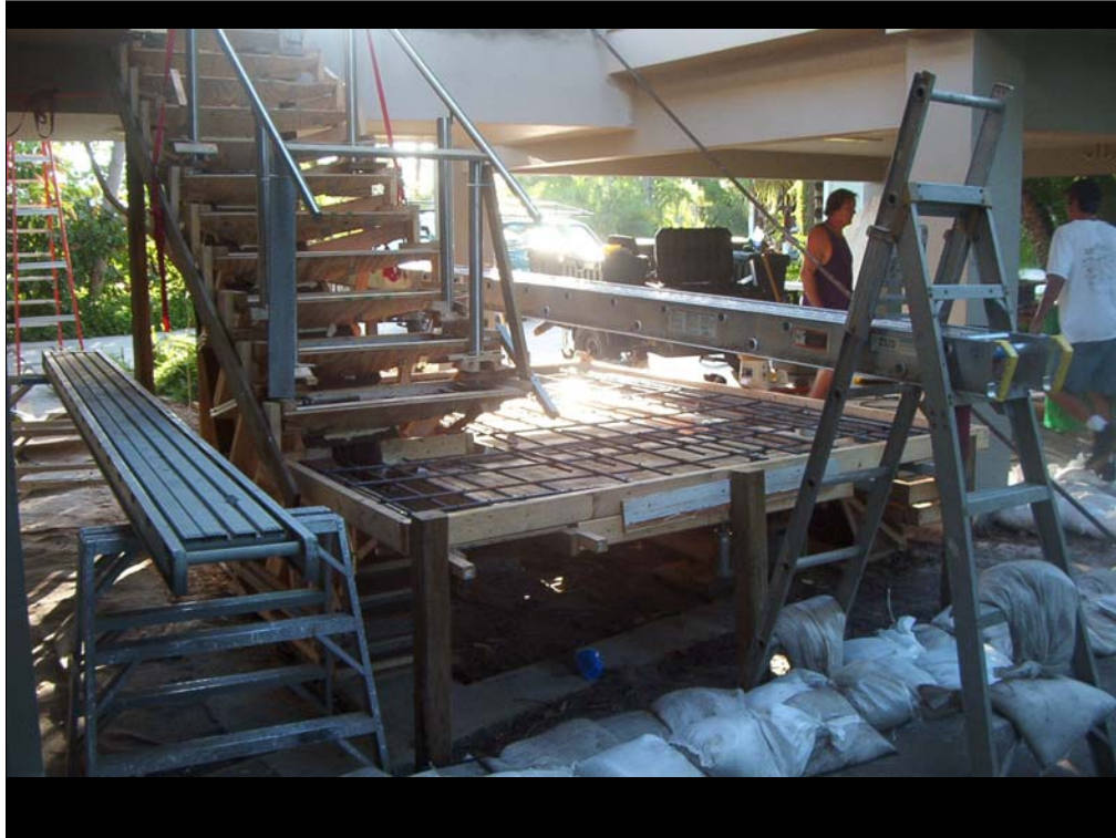
Tread boxes with rail verts in place.
