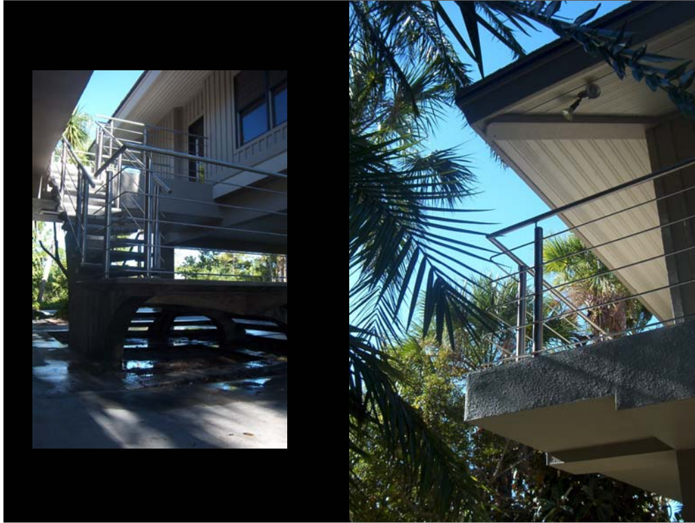
Corners in railings.
