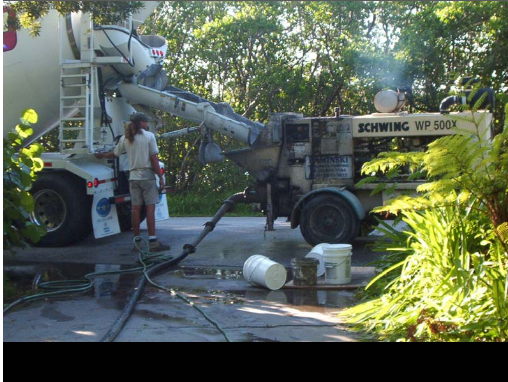
The ready mix truck (Dunco) and James's concrete pump – heavy duty hydraulic piston pump can handle the high cement content of the 5000psi mix. Danny in foreground waiting for the truck to mix in the Eucon WR75 water reducing admixture – buckets in foreground.
