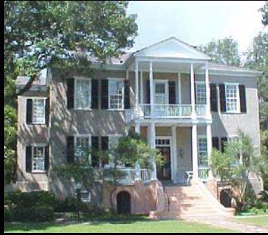
South Carolina: Tabby Manse (1211 Bay Street, Downtown Beaufort): Built by Thomas Fuller in 1786, the house has exterior tabby walls two feet thick (finished with stucco). Held by wooden pegs, its structural timbers measure twelve inches thick. Richard Fuller (1804-1876), the famous Baptist clergyman, was one of the builder's seven children.
