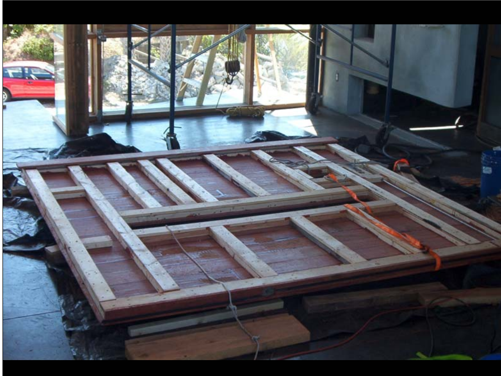
The door on its back face nearly ready for installation just after the hardware was installed in the frame.
