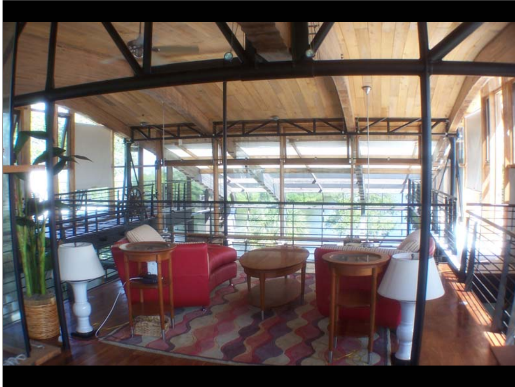
The 4 clerestory panels can be seen in the background just below the far pipe truss.
